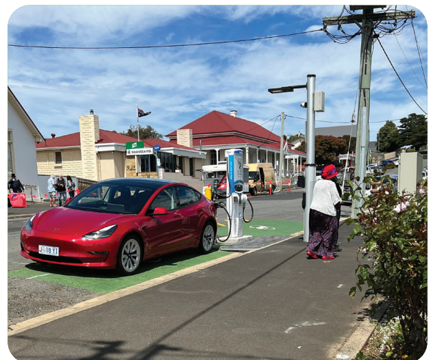
EV charging station. Noyes Street, Swansea
